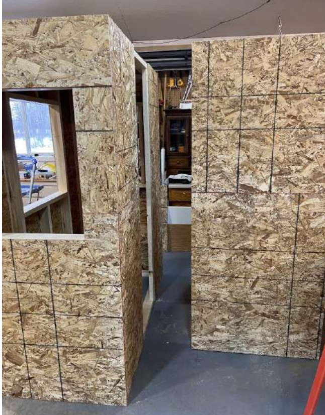
Figure 15 Basic Frame of Cabin Broken into Two Parts (main body on left and tail on right)
