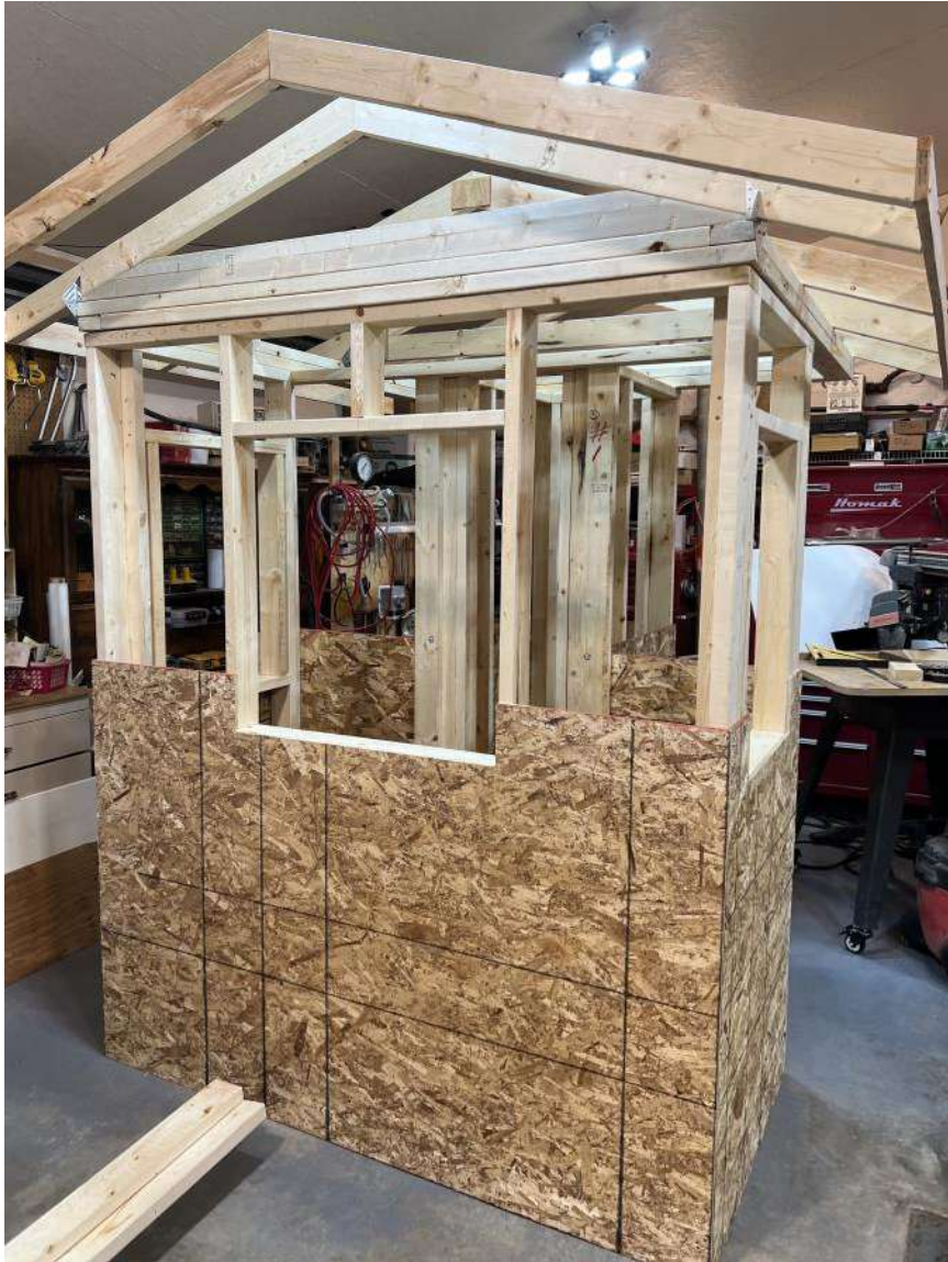
Figure 12 Basic Frame Common to All Cabins
