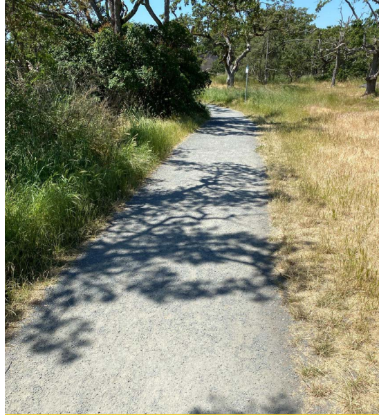
Non-combustible gravel on pathway
