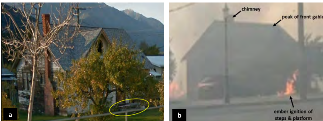
Figure 21: Burning embers ignited the ignition vulnerable wood steps and decking at the front entry way (a) of the house (a, yellow oval). Another ember ignited structure (b) is in the background to the left of the house in front. This house is also shown to the right of the Post Office in Figure 14.
