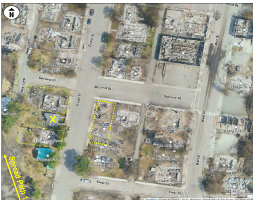
Figure 17: Post-fire Lytton Village scene between 1 and 3 Streets on July 12. The yellow X identifies the surviving house identified by a yellow arrow in Figure 14 (First Nations Emergency Services Society of BC).
