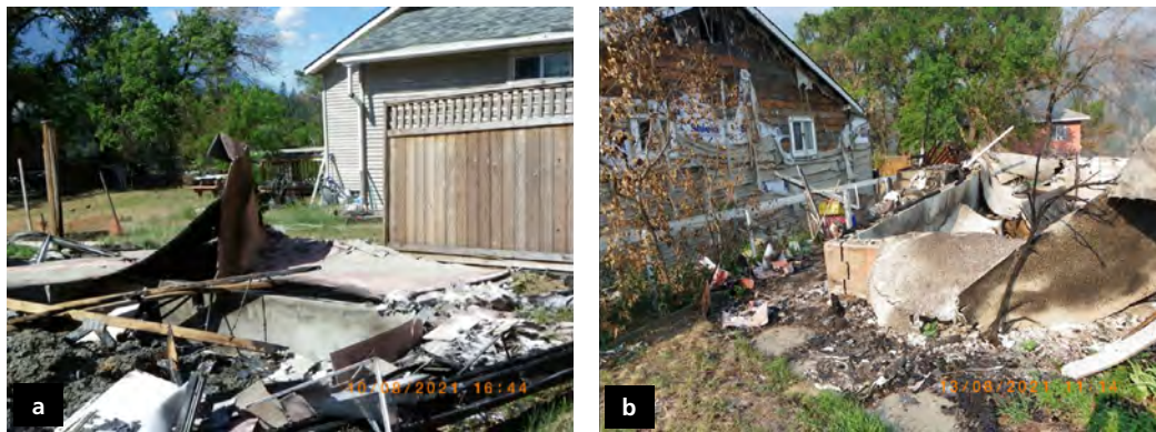
Figure 19: a, b) Adjacent burned houses to the south (left) and north (right) have non-flammable stucco exterior walls.
