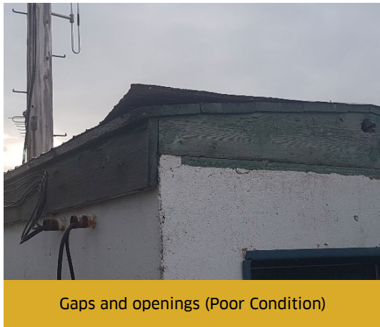
Figure 1. Example of class A rated (metal) roof in poor conditions with gaps and openings that allow ember penetration (left) and good condition (right), with no gaps or openings.
