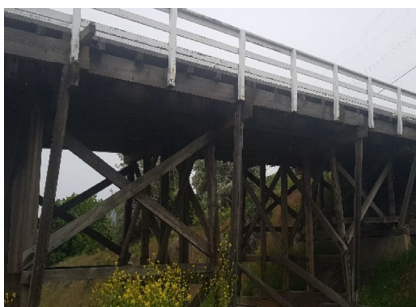
Figure 6. Example of bridge construction gaps and cracks where embers can penetrate and lodge
