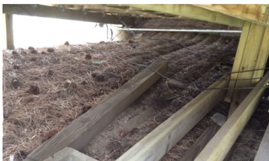
Open foundation with combustible debris
