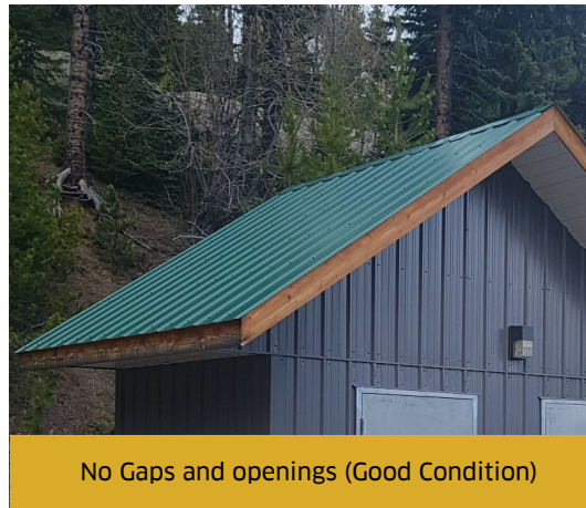
Figure 1. Example of class A rated (metal) roof in poor conditions with gaps and openings that allow ember penetration (left) and good condition (right), with no gaps or openings.
